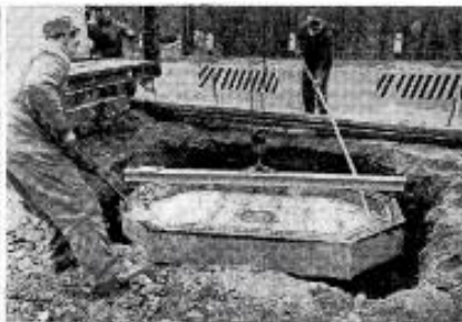
Lower manhole vault...
